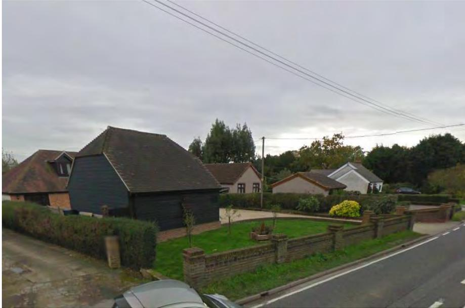
This property has a substantial brick boundary wall, approximately 0.75m to 1m back from the kerb face, the brick work does not match the rest of the wall and therefore appears to have been erected at a later date.
