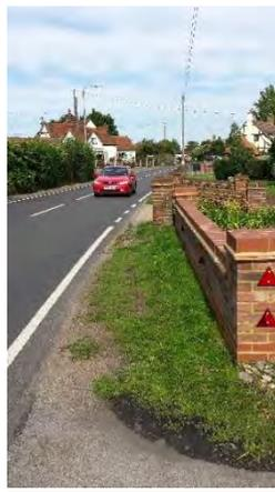
This wall is set back 1.3m from the carriageway and although this does provide a small refuge area for pedestrians this is below the recommended minimum width of 1.5m
