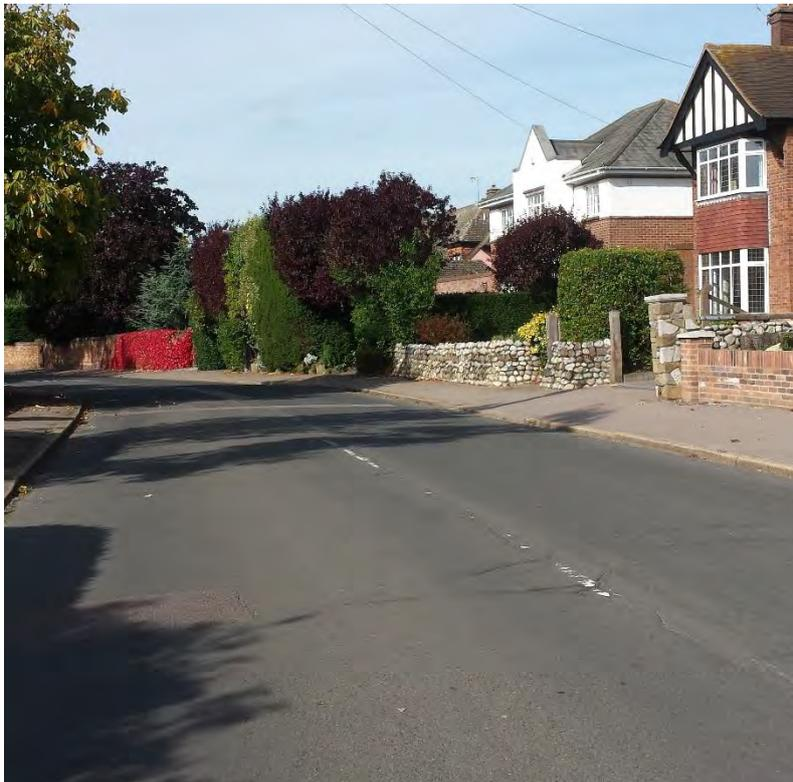
**Urban section – lane markings almost lost longitudinal and transverse cracking suggesting composite carriageway**
